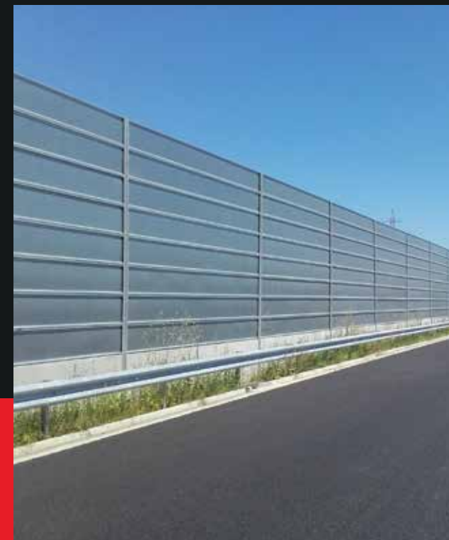
Sound Barrier Fencing
