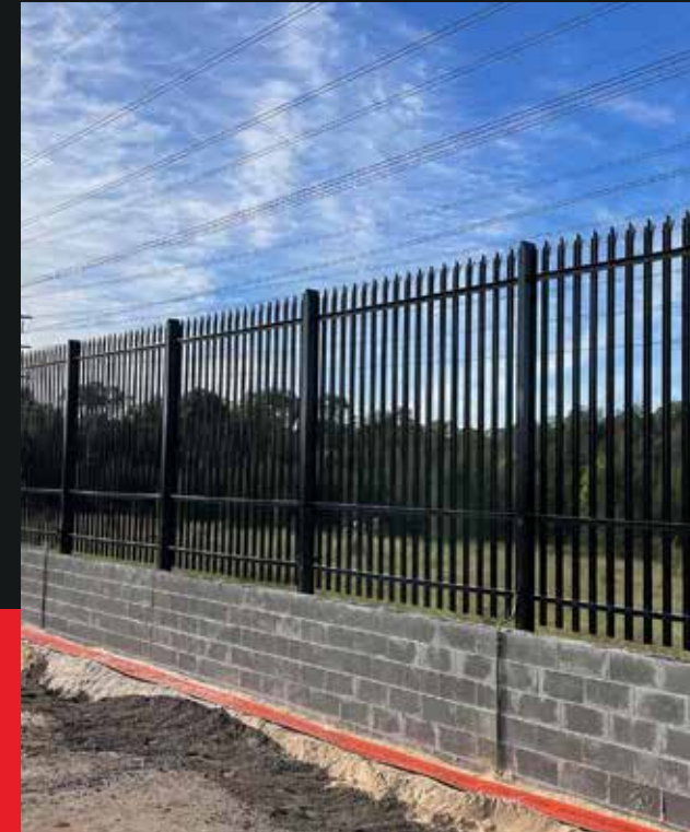
Steel Security Fencing
