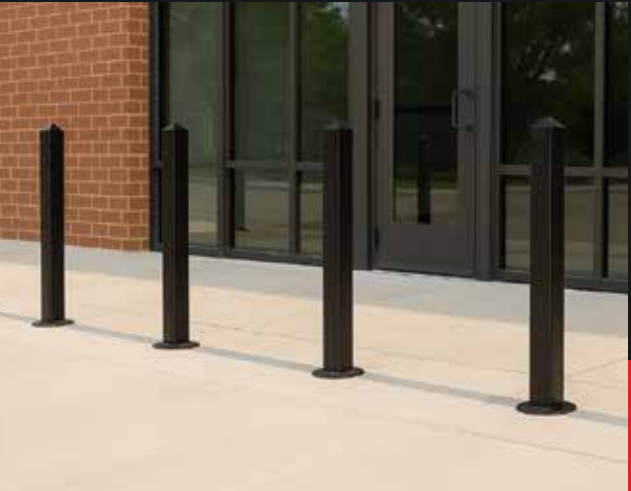
Embedded Steel Bollards
