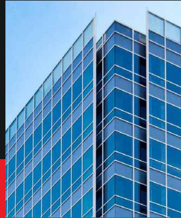
Spandrel Glass Panels
