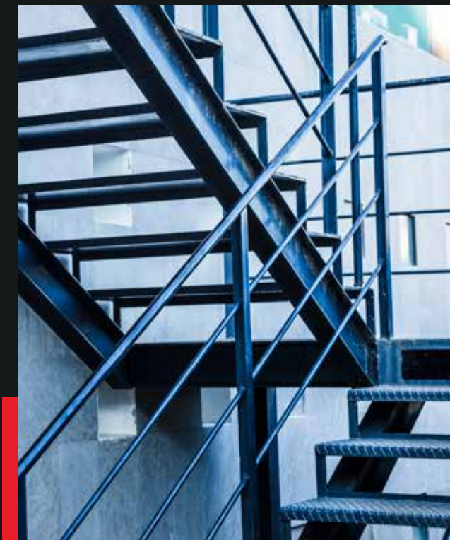
Emergency Exit Staircase
