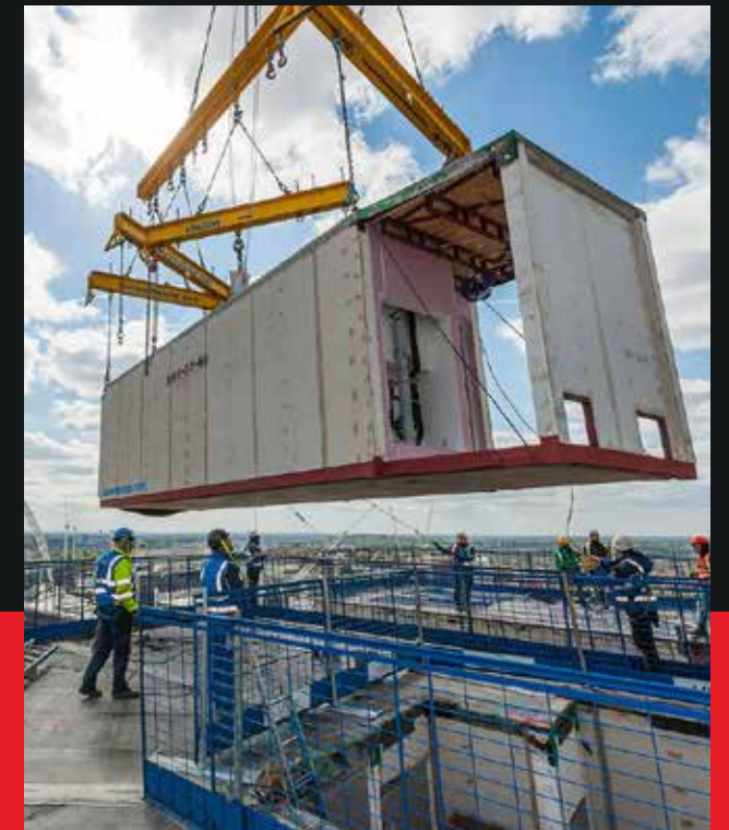
Prefabrication & Modular Fabrication
