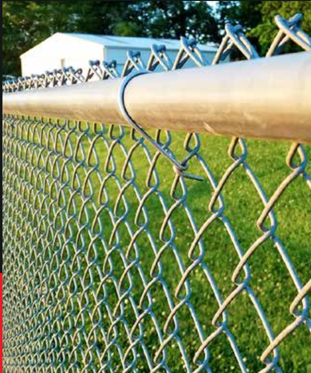
Galvanized and PVC-Coated Chain-Link Fencing
