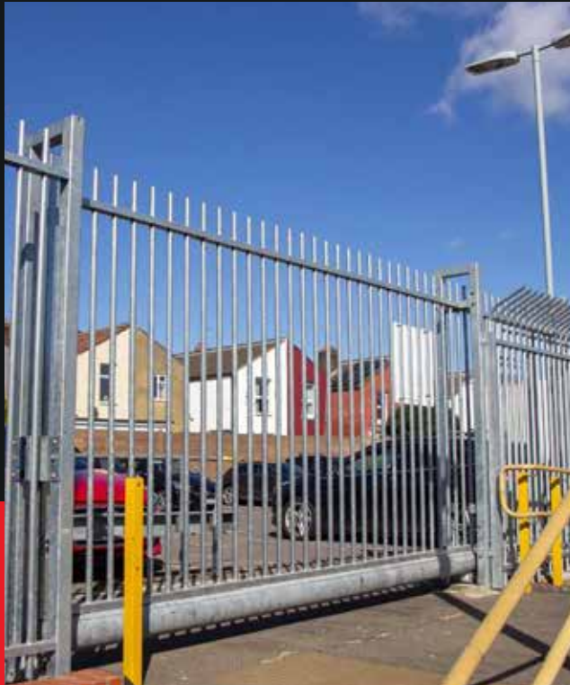
Railway Perimeter Fencing
