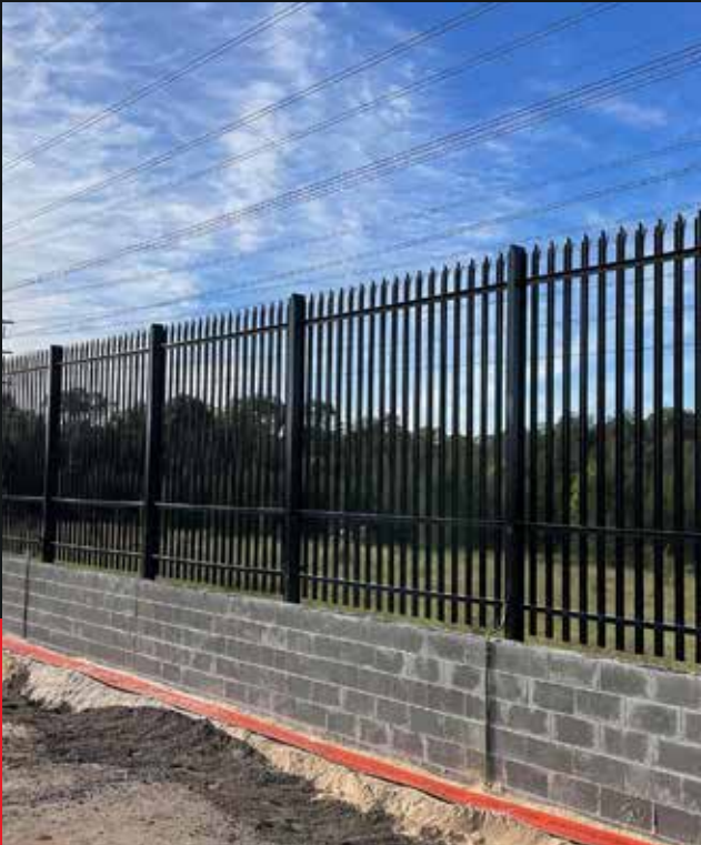
Steel Security Fencing
