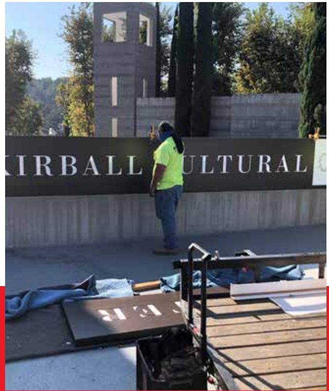
Signage Fabrication & Installation
