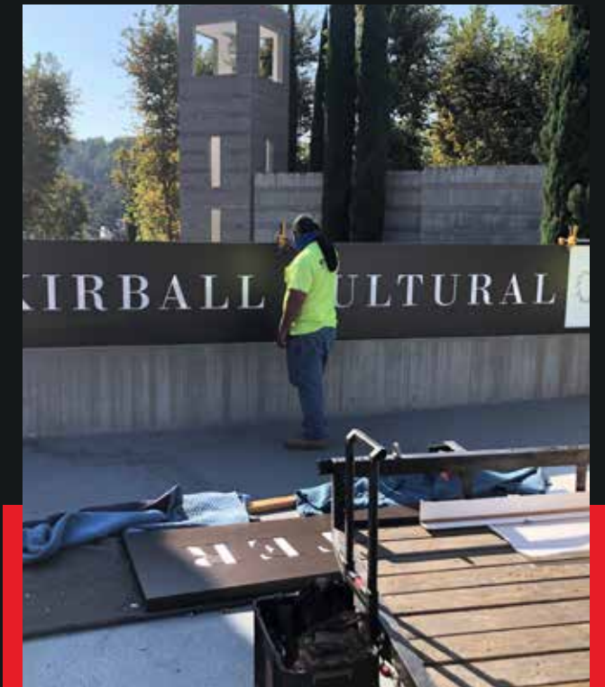
Signage Fabrication & Installation
