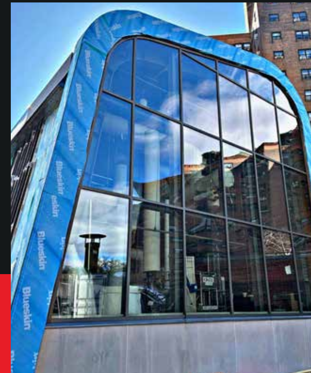
Architectural Metal & Glass Installation
