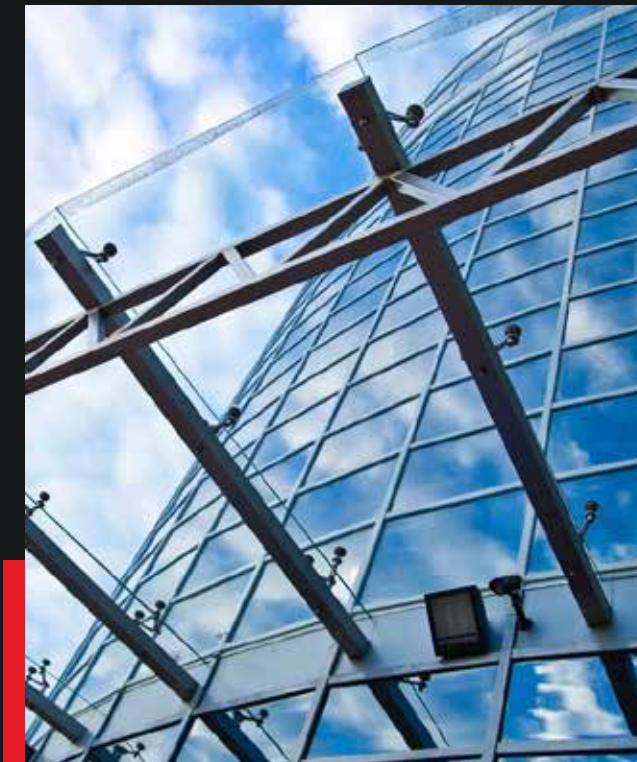
Spider-Fixed Glass Panels (Point-Fixed)
