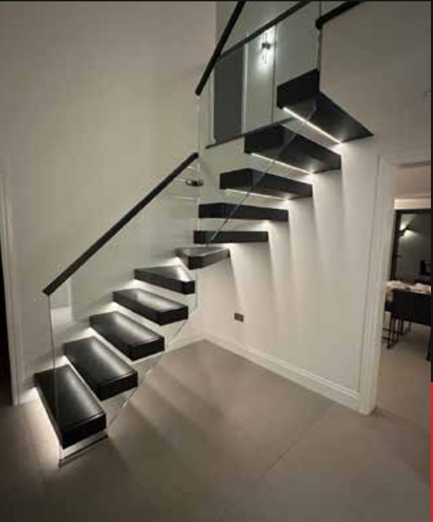
Cantilevered Floating Staircase
