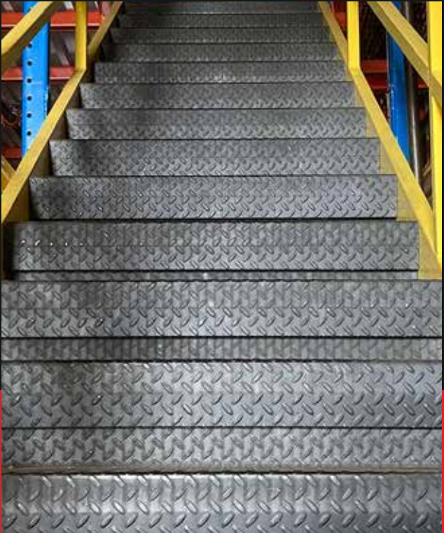
Checker Plate Staircase
