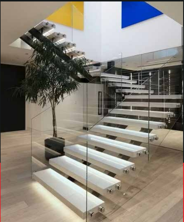
U-Shaped Staircase with Mid-Landing
