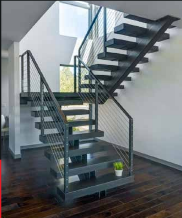
Half-Turn Staircase with Landing
