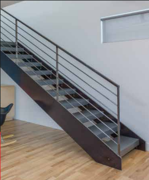
Open Riser L-Shaped Staircase
