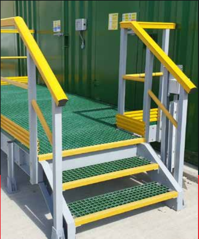
Utility Platform Staircase
