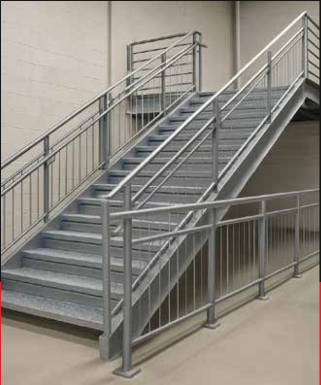
Split Straight Staircase (with landing)
