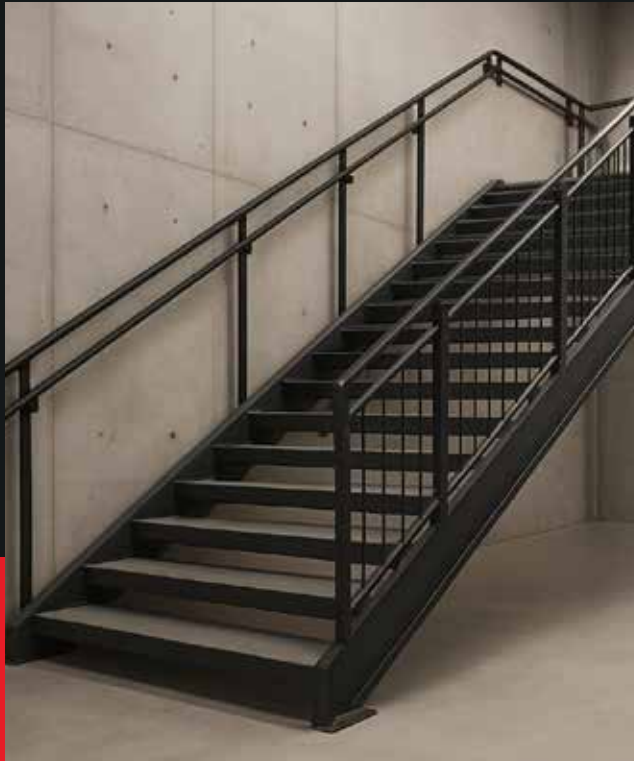
Open Riser Straight Staircase
