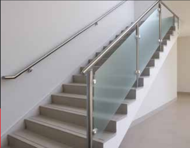
Glass Stair Guardrail
