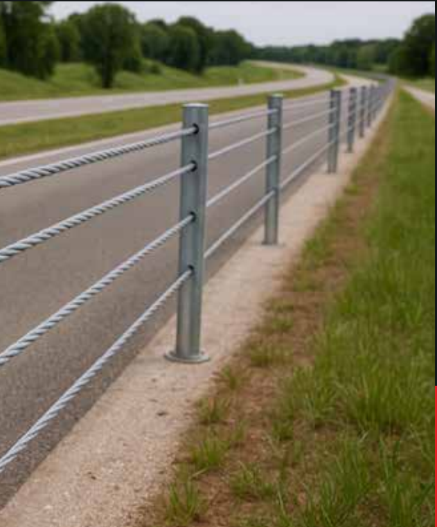
Cable Barrier Guardrail
