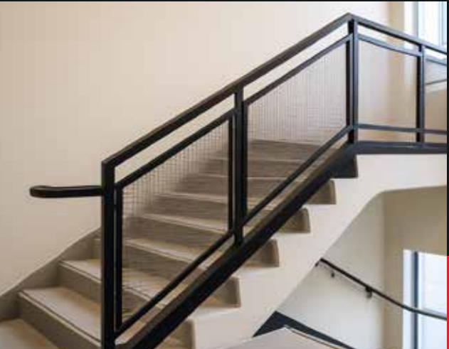
Mesh Stair Guardrail
