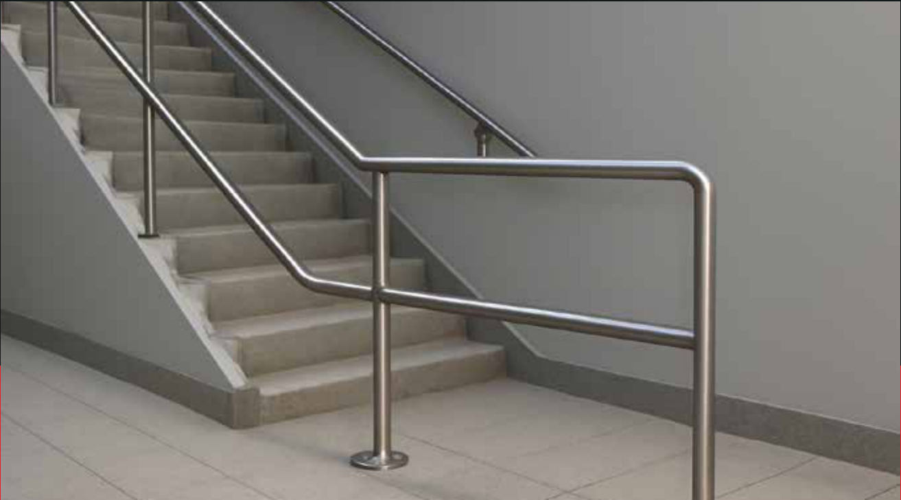
Double Rail Handrail
