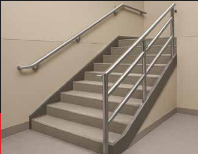
Standard Stair Guardrail
