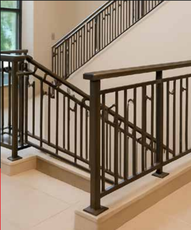
Decorative Stair Handrail
