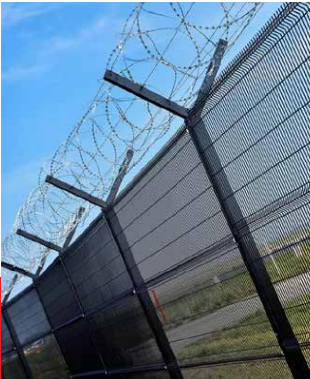
Perimeter Protection Fencing
