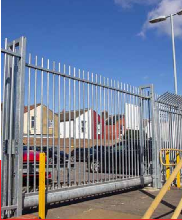
Railway Perimeter Fencing
