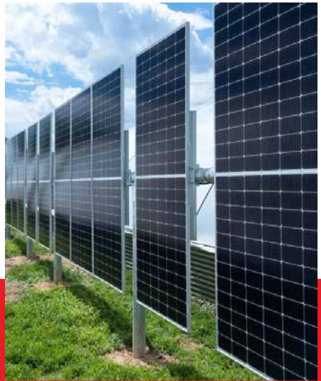
Solar Farm Security Fencing
