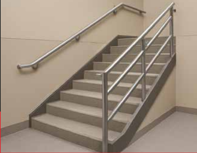
Standard Stair Guardrail
