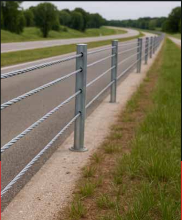
Cable Barrier Guardrail
