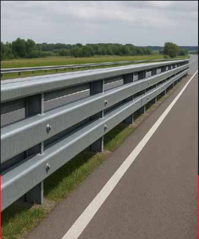
Box Beam Guardrail
