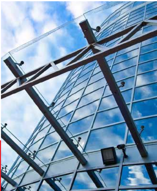
Spider-Fixed Glass Panels (Point-Fixed)
