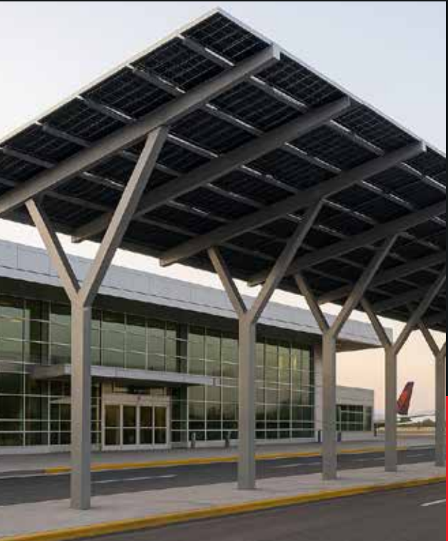
Solar Panel Canopies
