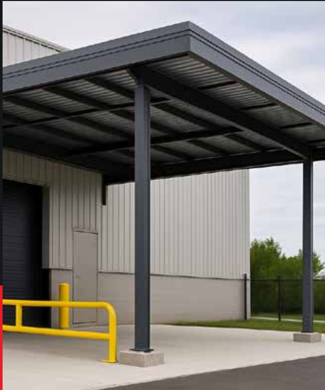
Loading Dock Canopies
