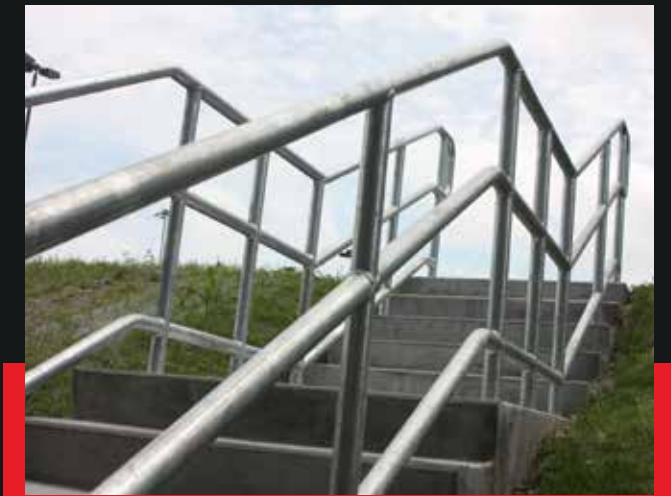
Galvanized Steel Railings
