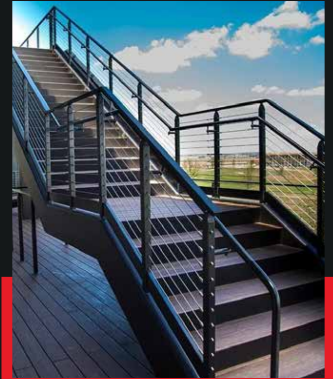
Double Rail Systems (Stair + Ramp)
