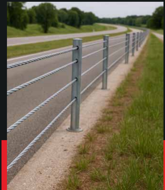
Cable Barrier Guardrail
