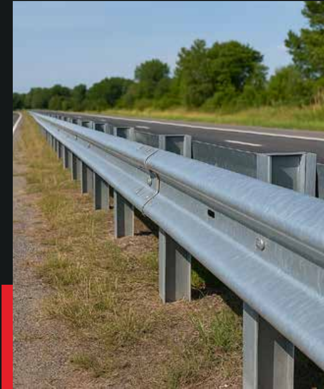
W-Beam Guardrail
