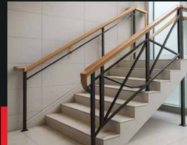
Custom Stair Guardrail
