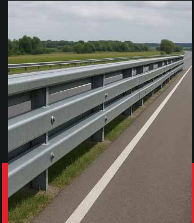
Box Beam Guardrail
