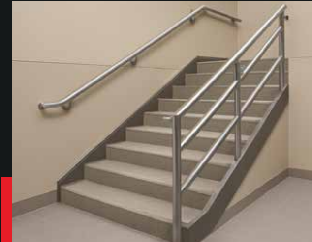
Standard Stair Guardrail
