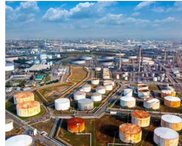
Oil and Gas: Pipeline supports and industrial equipment.
