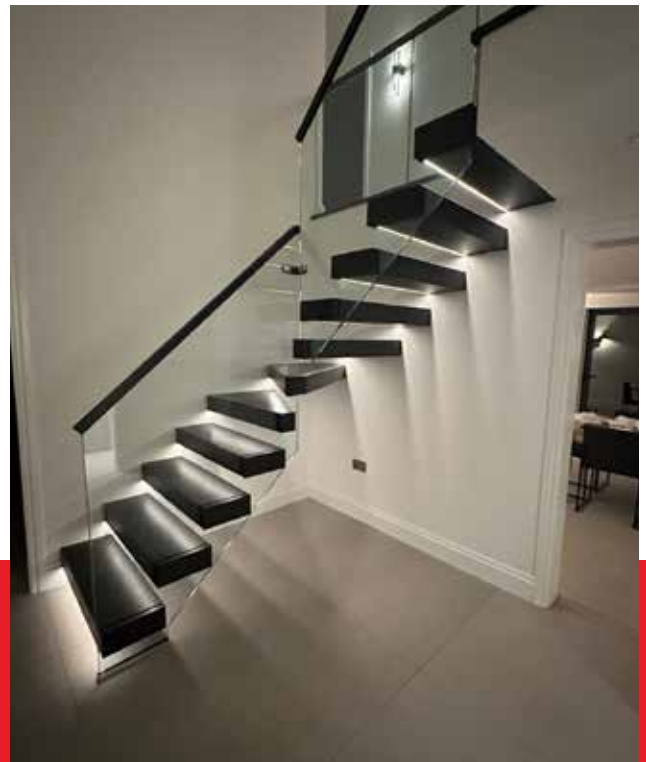
Cantilevered Floating Staircase
