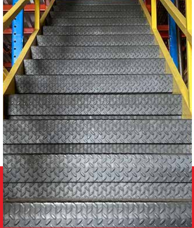
Checker Plate Staircase
