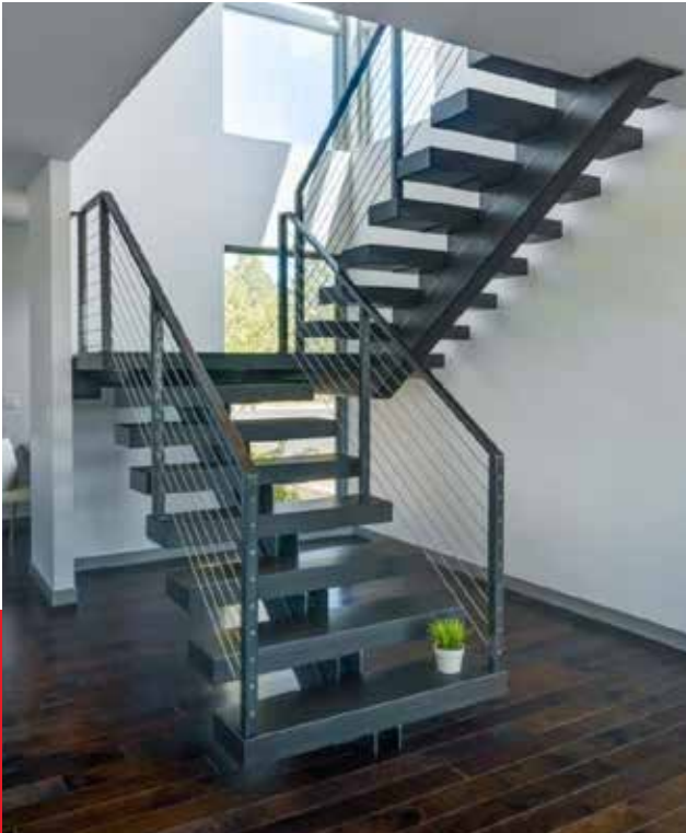
Half-Turn Staircase with Landing
