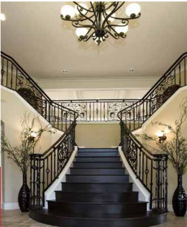
Split U-Shaped Staircase (grand entry)
