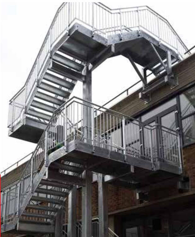
Square Spiral Staircase
