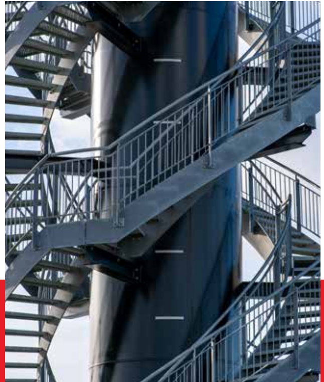
Double Helix Spiral Staircase
