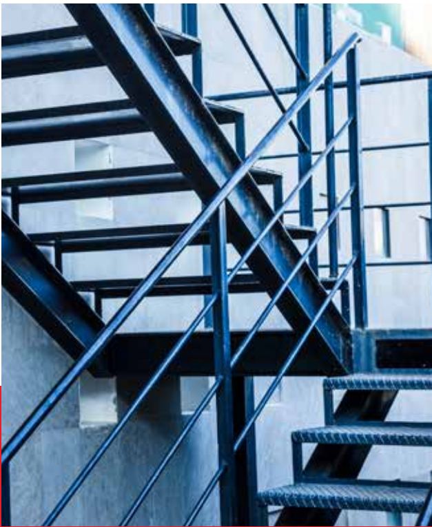
Emergency Exit Staircase
