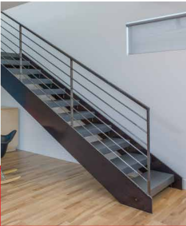
Open Riser L-Shaped Staircase
