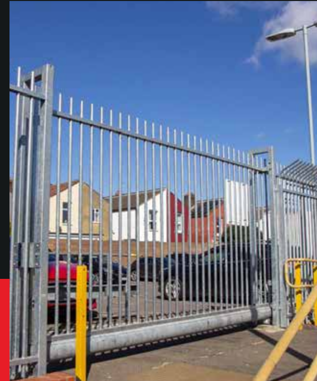
Railway Perimeter Fencing
