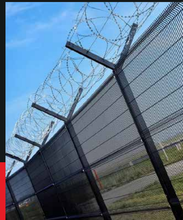
Perimeter Protection Fencing
