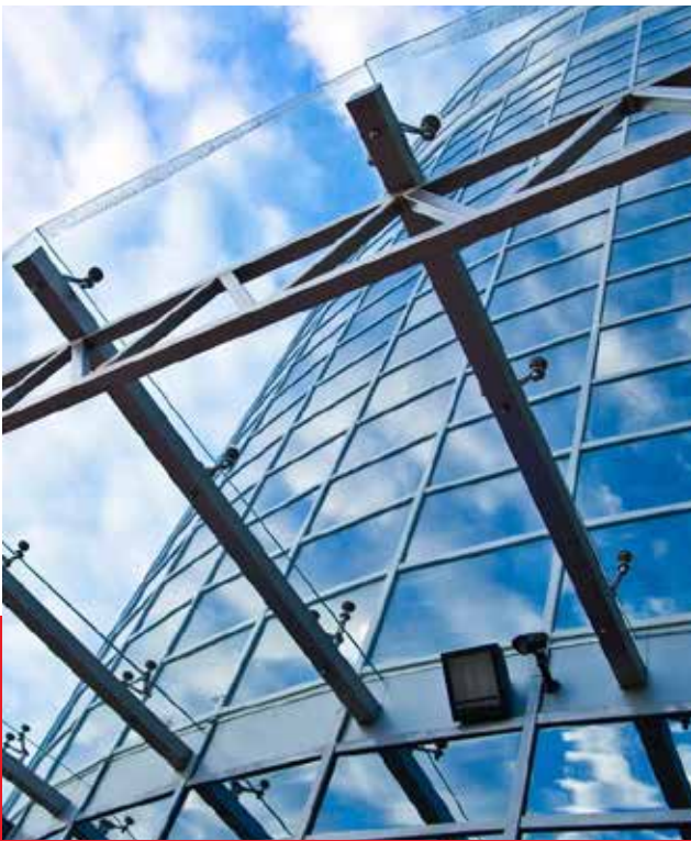
Spider-Fixed Glass Panels (Point-Fixed)
