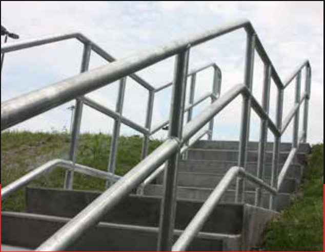
Galvanized Steel Railings
