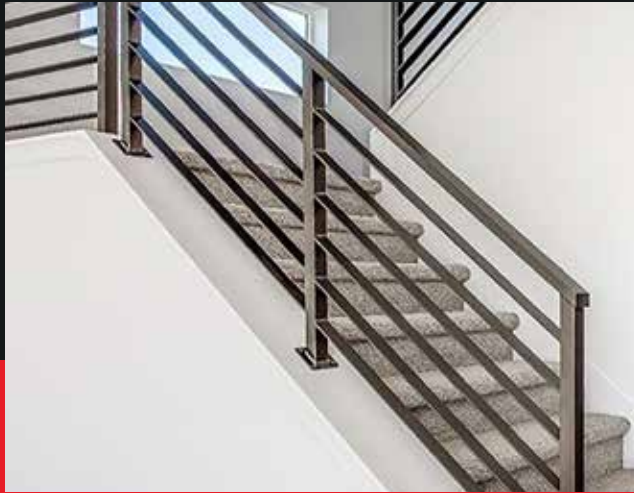
Mild Steel Pipe Railings
