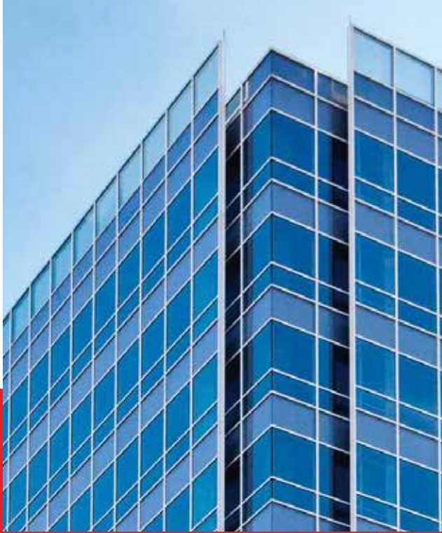
Spandrel Glass Panels
