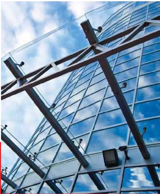
Spider-Fixed Glass Panels (Point-Fixed)
