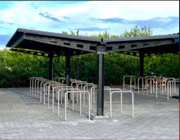
Double-Sided Covered Rack System
