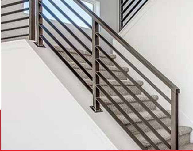
Mild Steel Pipe Railings
