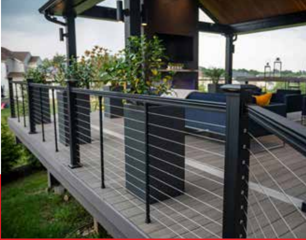
Powder-Coated Aluminum Railings
