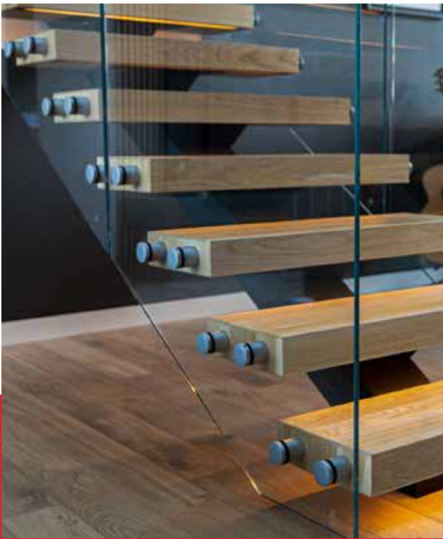
Standoff Mounted Glass Railings
