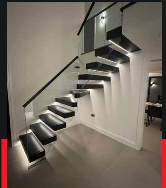
Cantilevered Floating Staircase
