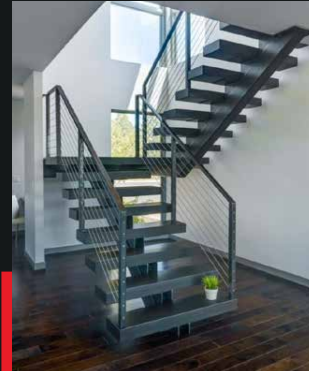
Half-Turn Staircase with Landing
