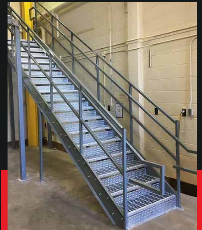
Closed Riser L-Shaped Staircase
