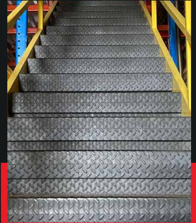
Checker Plate Staircase
