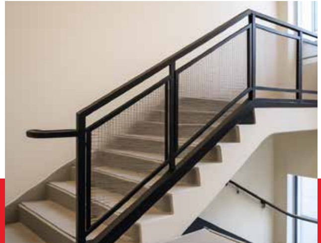
Mesh Stair Guardrail
