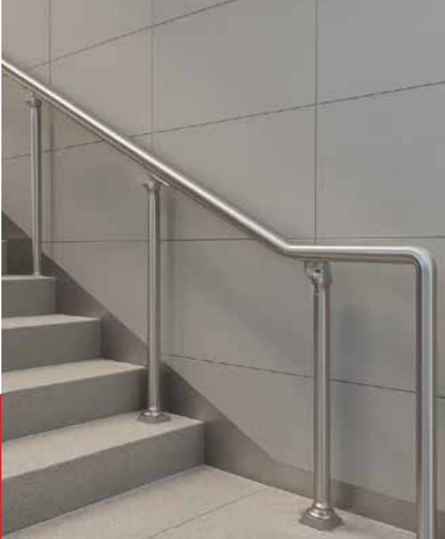
Standard Stair Handrail
