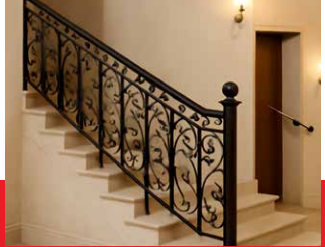
Decorative Stair Guardrail
