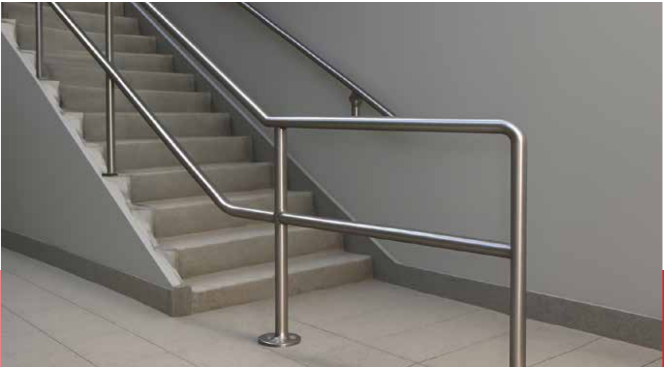
Double Rail Handrail
