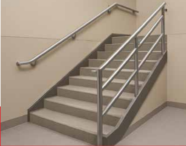
Standard Stair Guardrail
