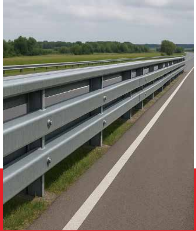
Box Beam Guardrail
