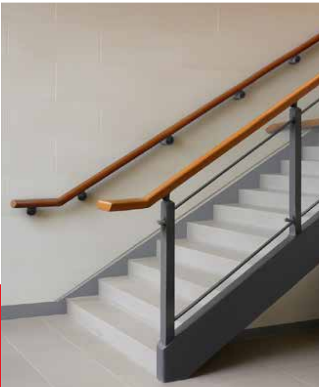
Custom Stair Handrail
