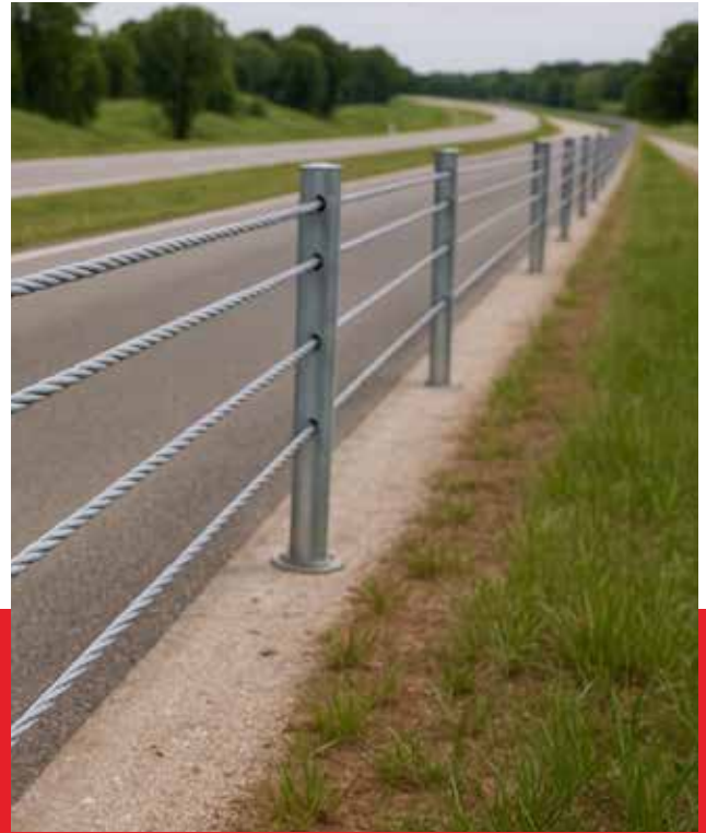
Cable Barrier Guardrail
