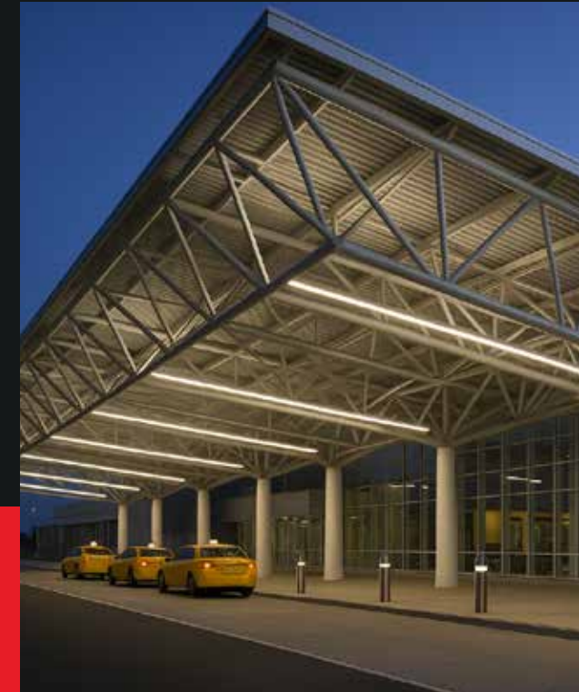
Structural Steel Canopies
