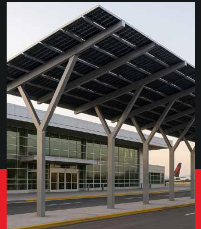
Solar Panel Canopies
