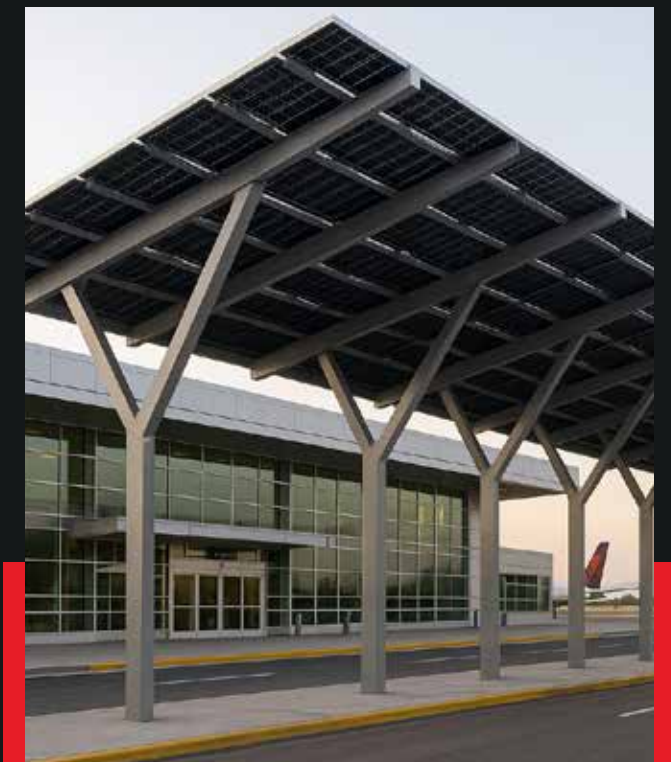
Solar Panel Canopies
