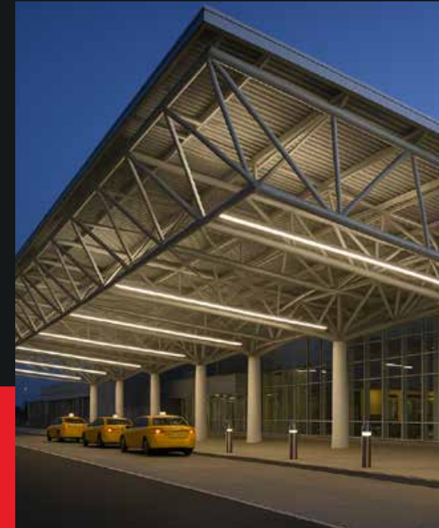
Structural Steel Canopies
