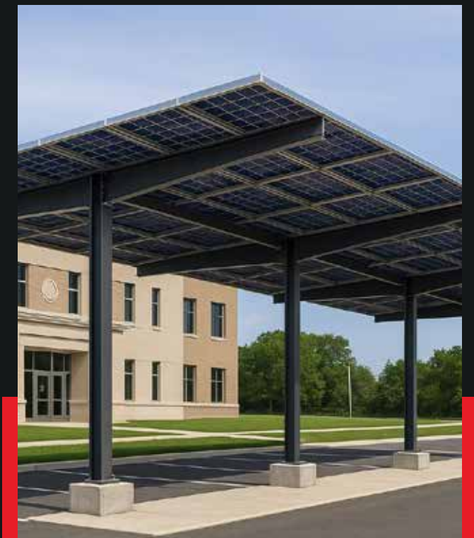
Solar Panel Canopies
