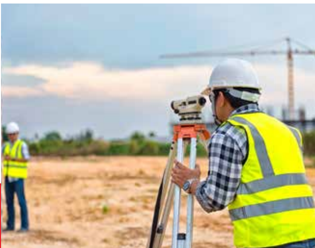
Topographic & Structural Survey
