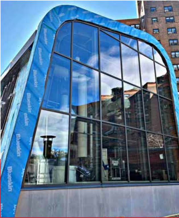
Architectural Metal & Glass Installation
