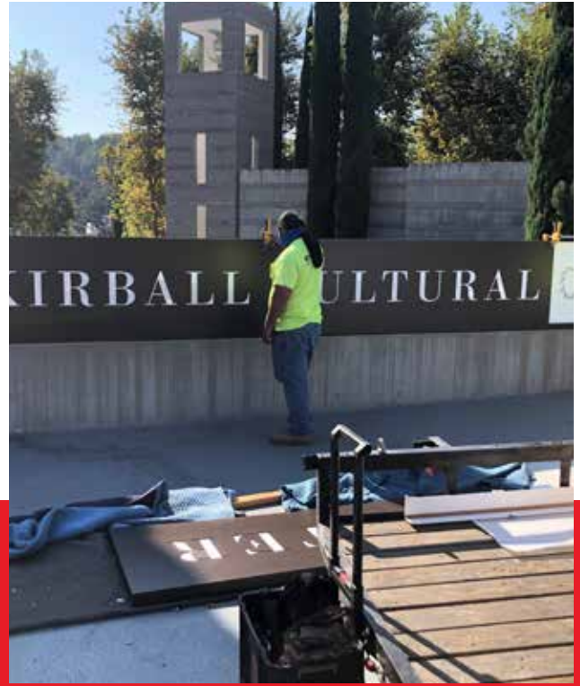
Signage Fabrication & Installation
