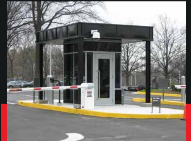
Surveillance Integrated Booth
