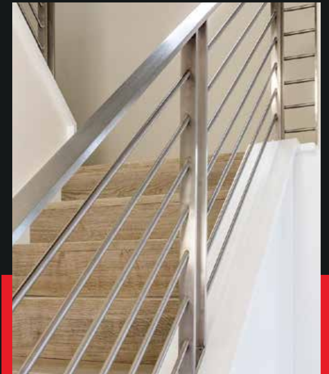
Brushed Finish Railings
