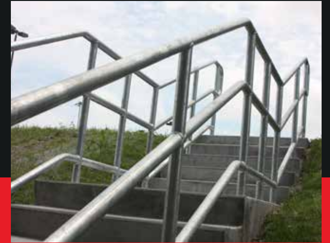
Galvanized Steel Railings
